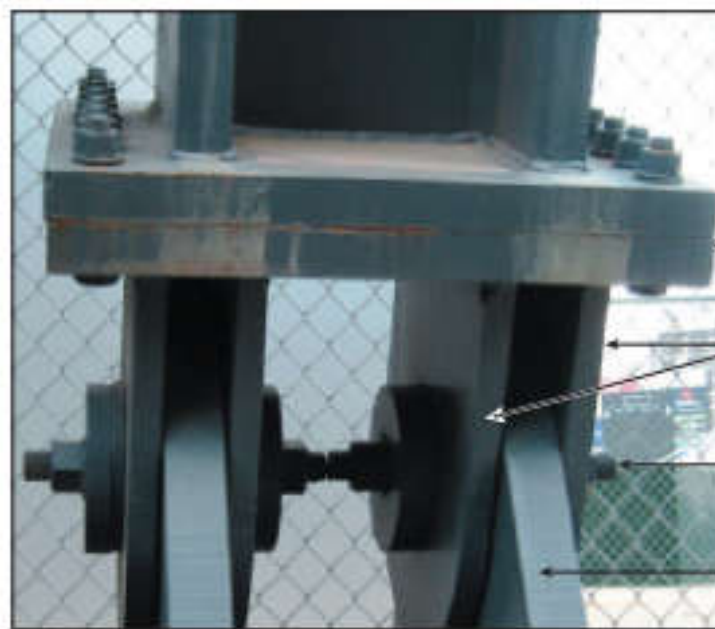
(b) Detail at bottom of brace (© Barry Goodno)
