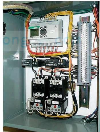
PLC-based control panel
